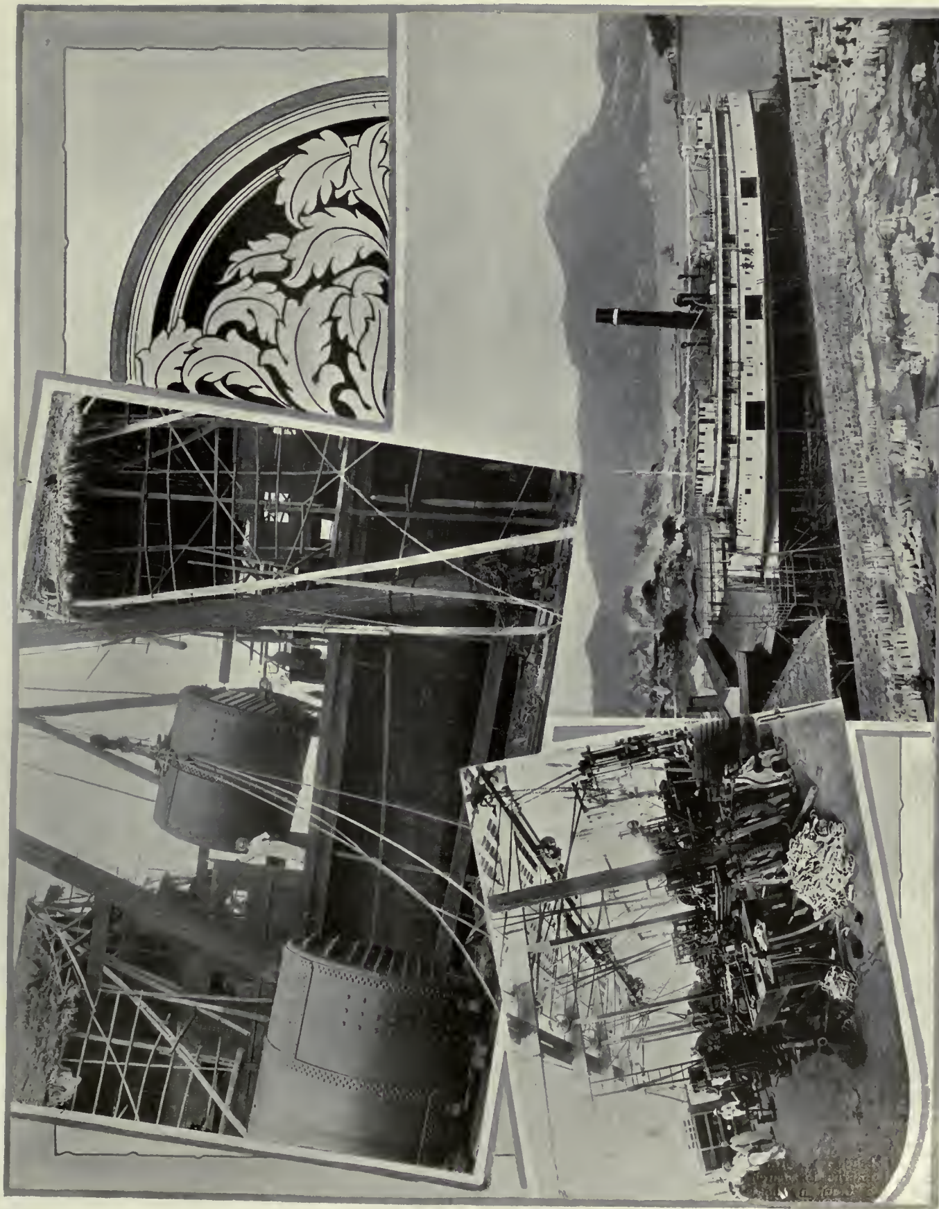
LIFTING IN THE "KWONG TUNG'S" BOILERS. VIEW OF MACHINE SHOP.
